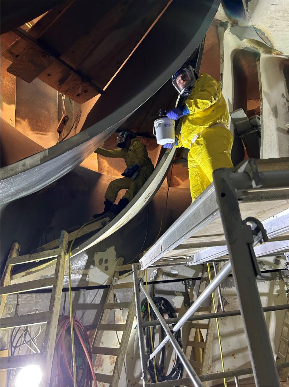
Figure 7.—Application of PE2 to Blade 7.
