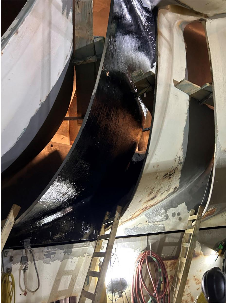
Figure 8.—Blade 7 shown coated with PE2.
