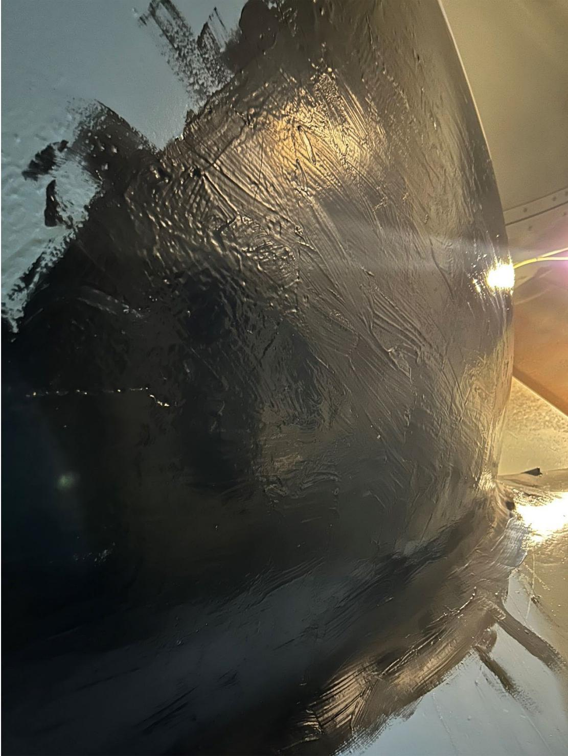
Figure 10.—The cavitation zone of Blade 8 shown coated with solvent-borne epoxy and PE2.
