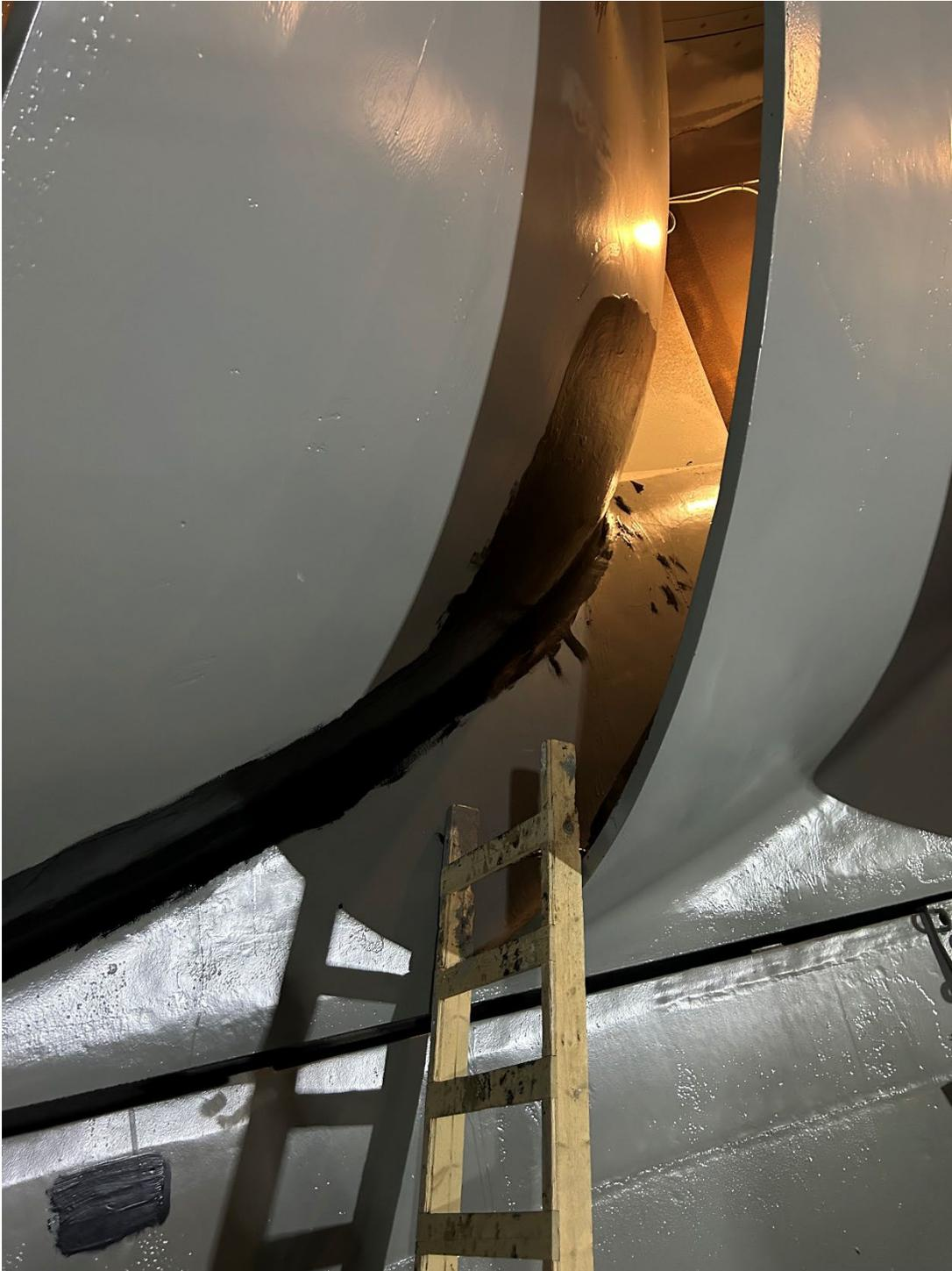
Figure 9.—The cavitation zone of Blade 8 shown coated with solvent-borne epoxy and PE2.
